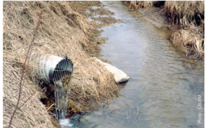
*Some agricultural soils retain too much water. Drainage is therefore carried out using perforated pipes in the ground. The underground pipes can more quickly evacuate water that seeps into the ground during spring thaws or heavy rains.*
